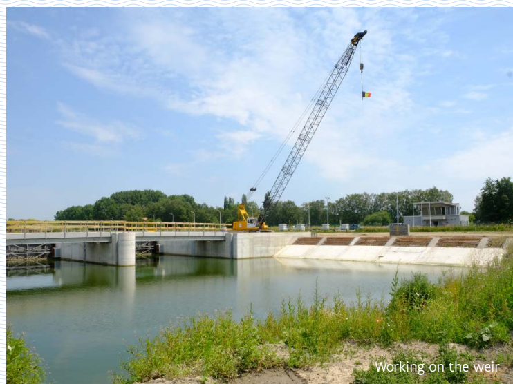
Installing weir segments
